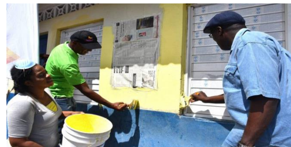
Figure 3: Renovation of Allman Town Primary School
