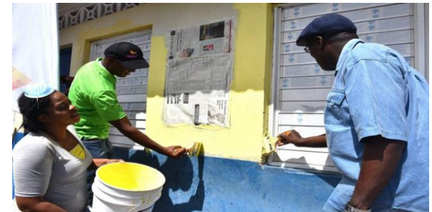
Figure 3: Renovation of Allman Town Primary School
